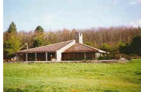
Hoh Tribal Center, Forks, WA
